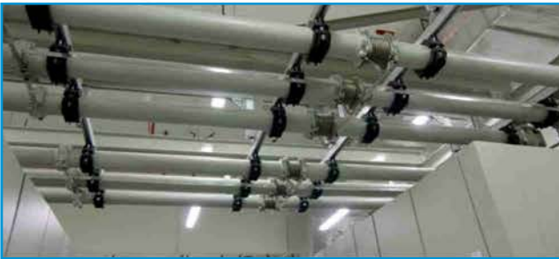
GASLINK® SF 6 insulated busbar system
