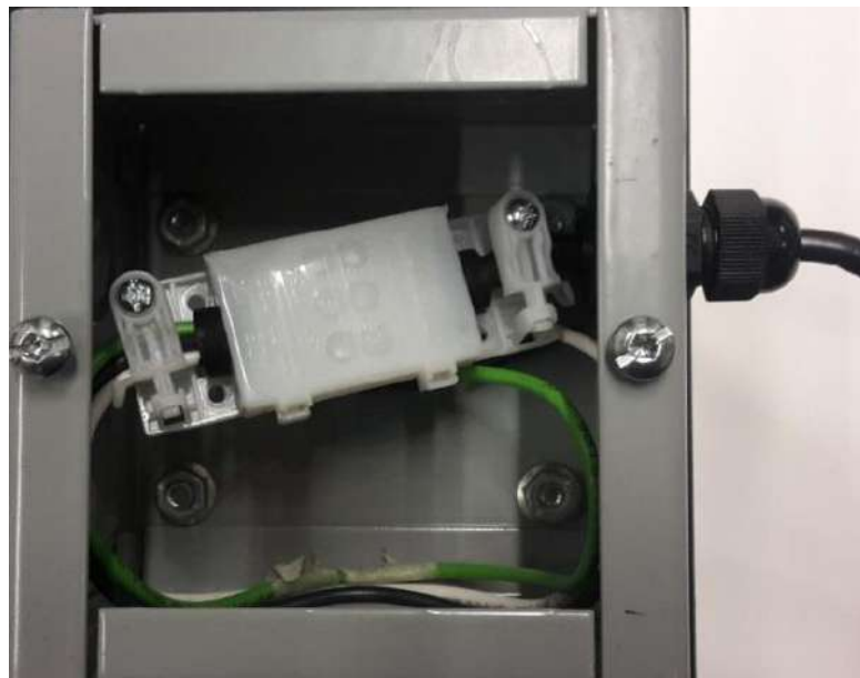
Fig. 40 Completed electrical connections to the projector 74-00013-01
